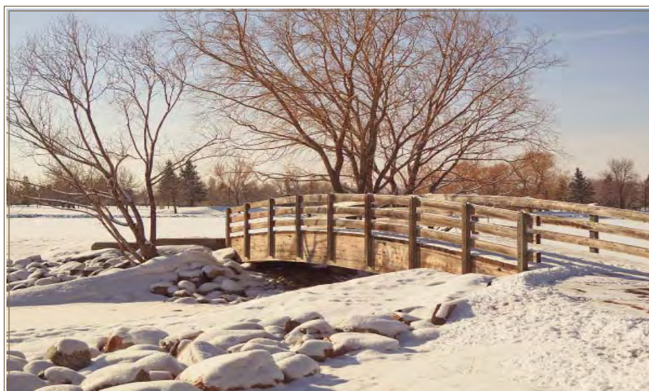
Pathway Bridge at Henderson Lake
