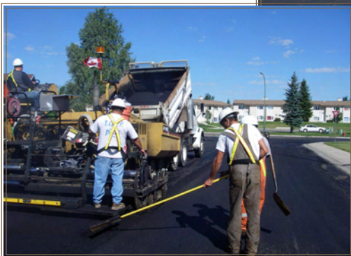
Paving Ryerson Road West Columbia Boulevard to Trent Road West
