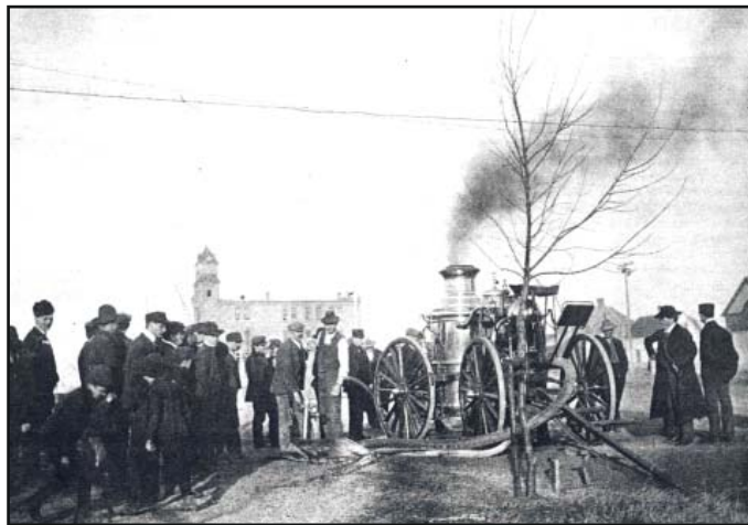
1985 Ronald Steam Engine pumping water from an underground tank in the square
