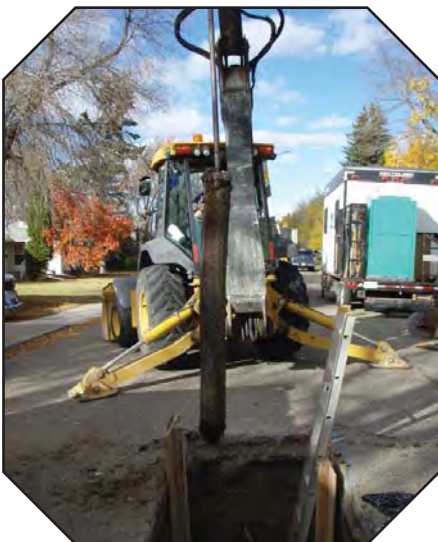
Removing roots from riser
