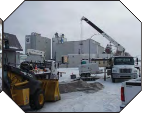
Installing an 18 " butterfly valve to upgrade the water distribution system 1200 block. 2 Avenue S
