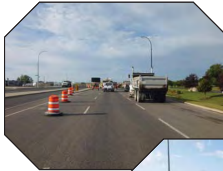
Top lift of asphalt on all four lanes
