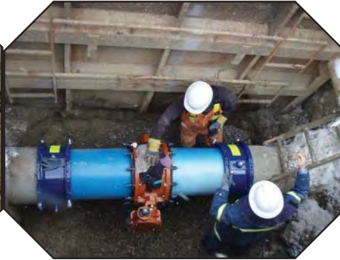
Installing an 18 " butterfly valve to upgrade the water distribution system 1200 block. 2 Avenue S
