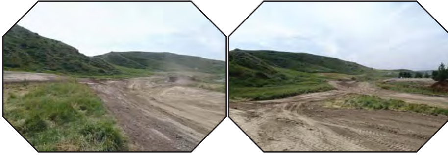
Extended view of drainage construction opposite to Soft Ball field.
