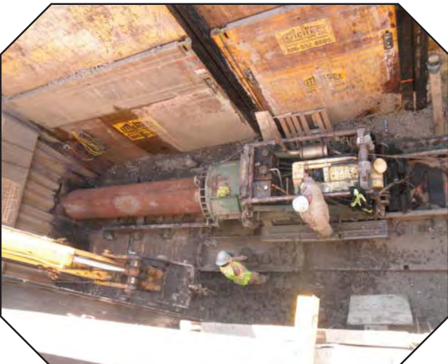
Guided auger boring a 18" sanitary main under 2A Avenue North
