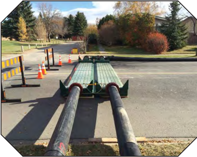
Sewer bypass pipes crossing 23rd Street North during sewer lining
