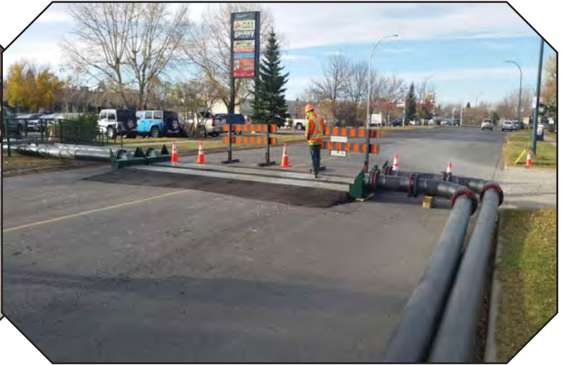
Sewer bypass pipes crossing 23rd Street North during sewer lining
