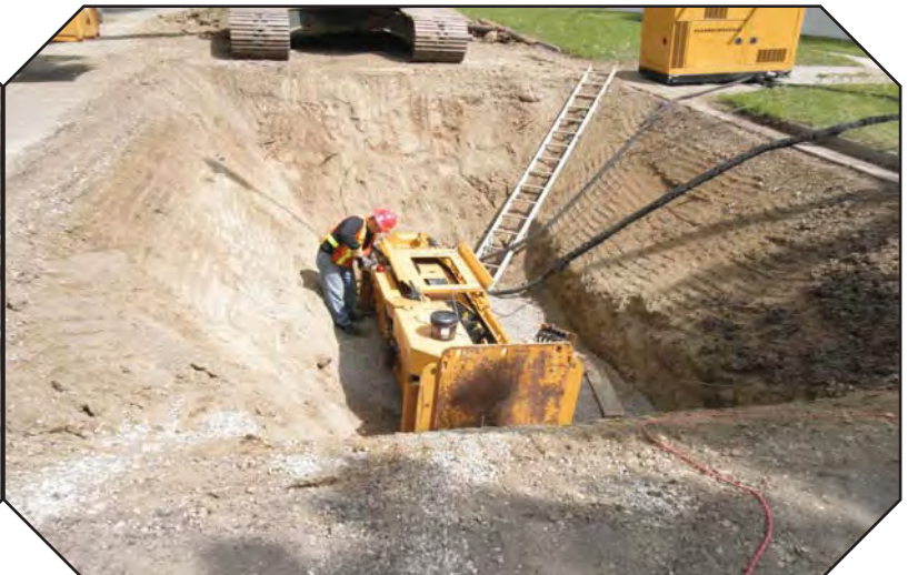
Preparation of static pipe bursting machine for 8A Avenue South watermain renewal
