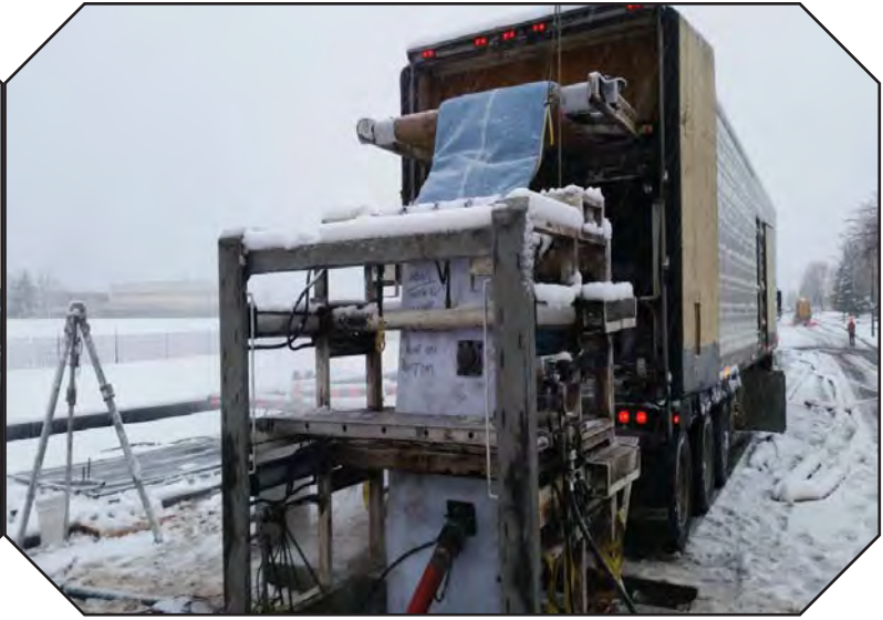
Liner being installed underneath 18th Avenue
