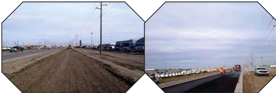
43rd Street North east lane, showing placing and rolling of asphalt.
