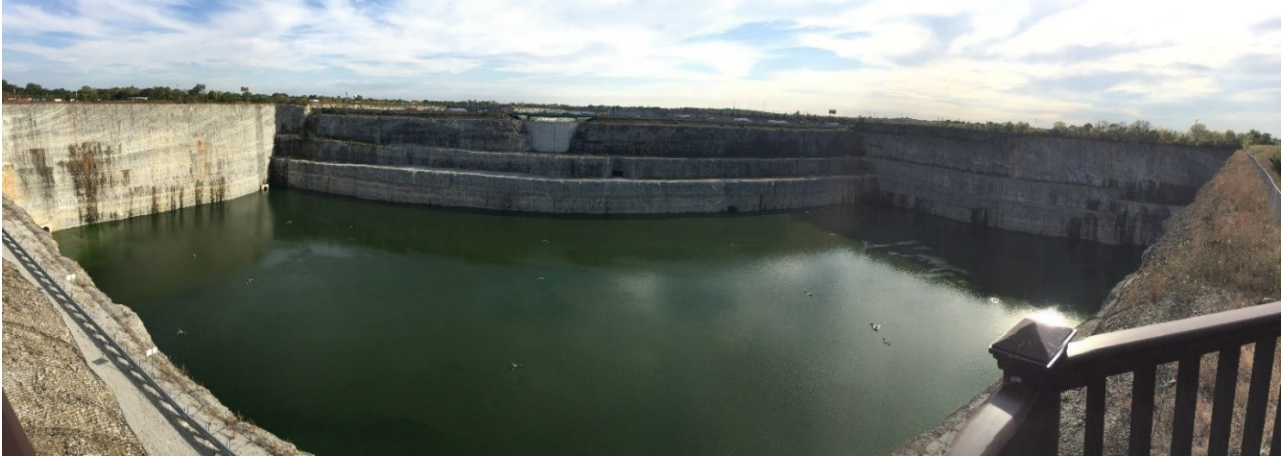
FIGURE 2.4 Thornton Quarry, the reservoir for TARP, outside of Chicago. SOURCE: Photo courtesy of Lauren Alexander Augustine, National Academies.
