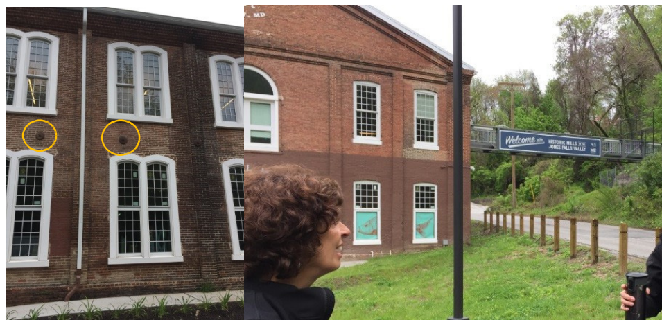
FIGURE 2.1 (Left) Image of newly renovated apartments inside a historic building. Rivets (circled in yellow) between the first and second floor windows mark the flood stage for this building. (Right) Image of newly renovated apartment building that includes an escape bridge on the second floor for safe egress during flooding. SOURCE: Photo courtesy of Lauren Alexander Augustine, National Academies of Sciences, Engineering, and Medicine.
