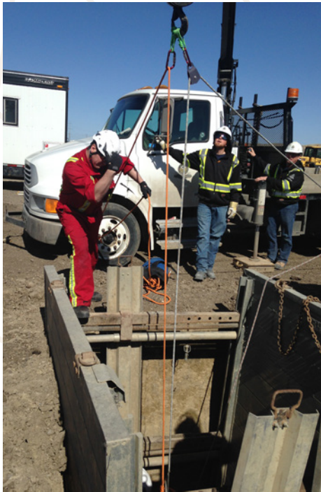
Water Main Replacement
