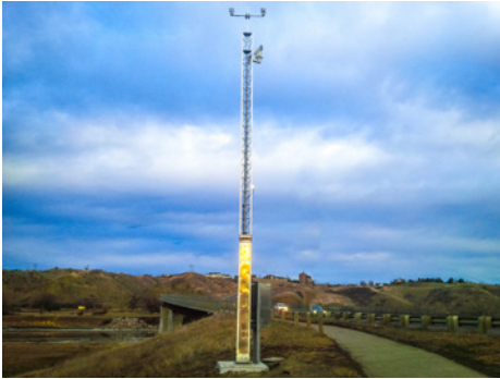
Whoop Up Drive RWIS Installation
