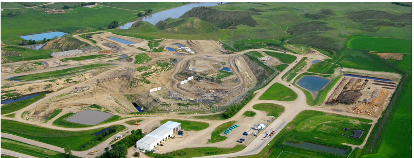
Waste and Recycling Aerial View
