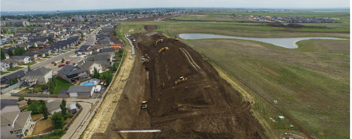
Metis Trail Sewer Installation
