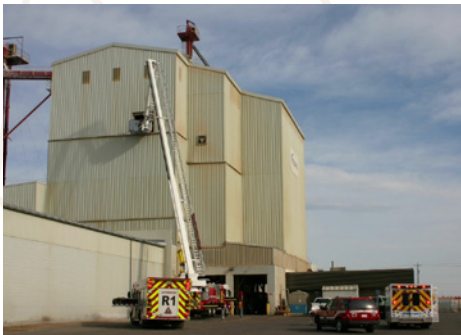
Rescue Operations at Viterra Elevator
