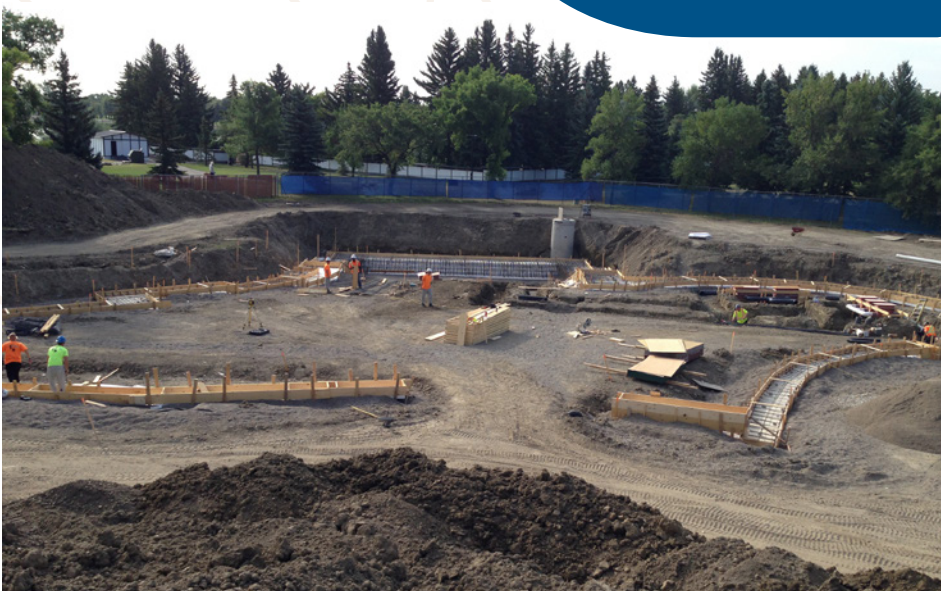
Henderson Outdoor Pool construction
