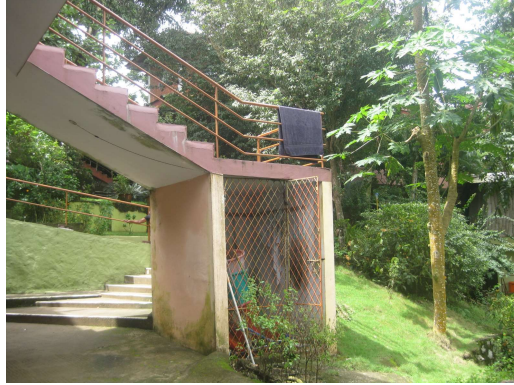
Figure 15 Shanti's new closet (picture taken August 2013)
