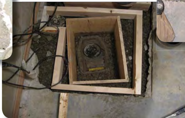
High water table before, mainline clean-out and weeping tile trap, and the after, new sump pump and mainline backwater valve as well as a normal closed valve on the floor drain
