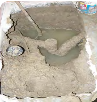
High water table before, mainline clean-out and weeping tile trap, and the after, new sump pump and mainline backwater valve as well as a normal closed valve on the floor drain
