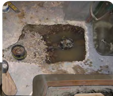
High water table before, mainline clean-out and weeping tile trap, and the after, new sump pump and mainline backwater valve as well as a normal closed valve on the floor drain
