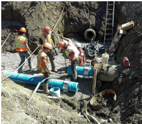
Mayor Magrath Drive Reservoir Piping Upgrades
