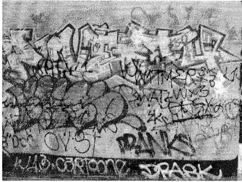
Figure 94. Graffiti covers a mural in one of the MacArthur Park tunnels.
