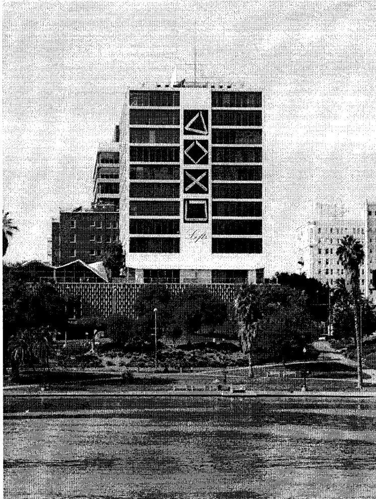
Figure 14. American Cement Building.
